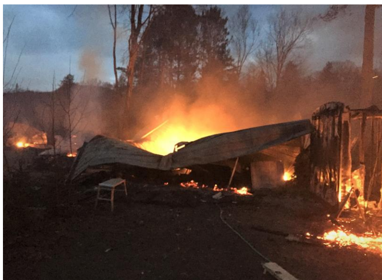
Figure 2: Fire completely consumes core processing facility
